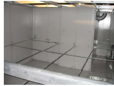
Photo Far Left: Internal View of Tank & Fittings
