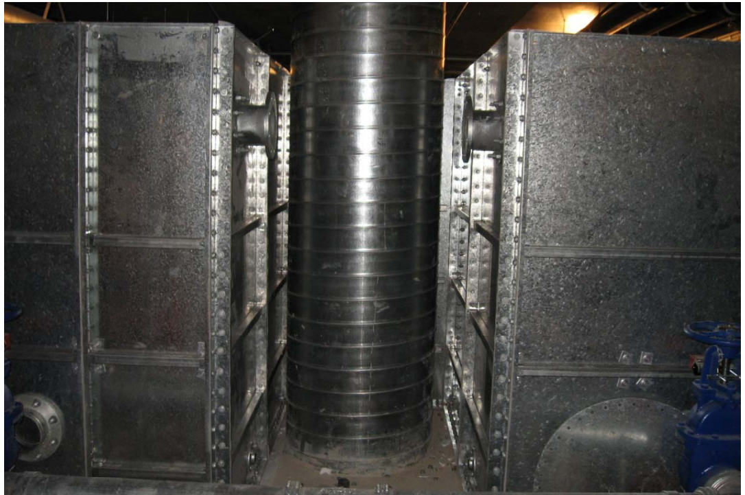
Photo Above: Completed TS250 Panel tank built around existing column
