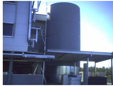
Photo Left: Insulated Tank in process of construction
